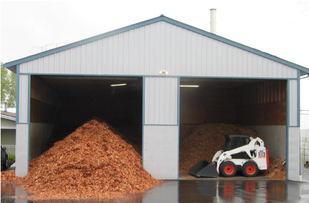
Waste wood heating system, wood storage, boiler room.
